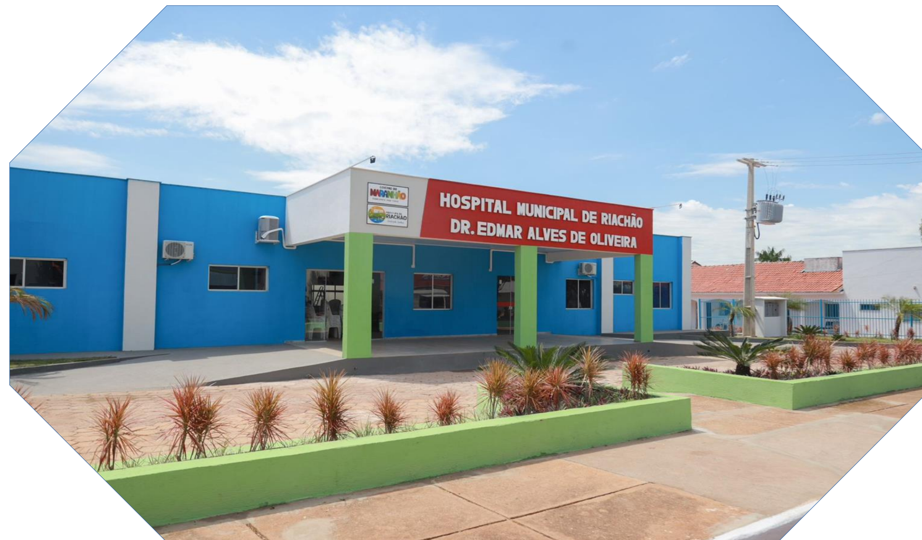
Reforma do Hospital Municipal de Riachão
